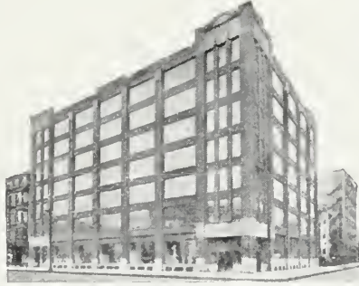
THE PAIDAR FACTORY
